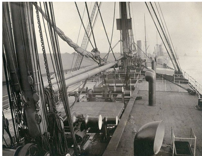
Californian, foredeck view showing deck winches that could adjust Californian alongside Titanic Credit: Flickr
